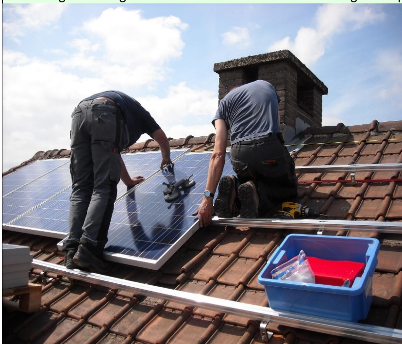
Fig. 8: Installing solar panels. Source: pixabay.com
